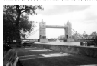
Tower Bridge (foto:autor)
